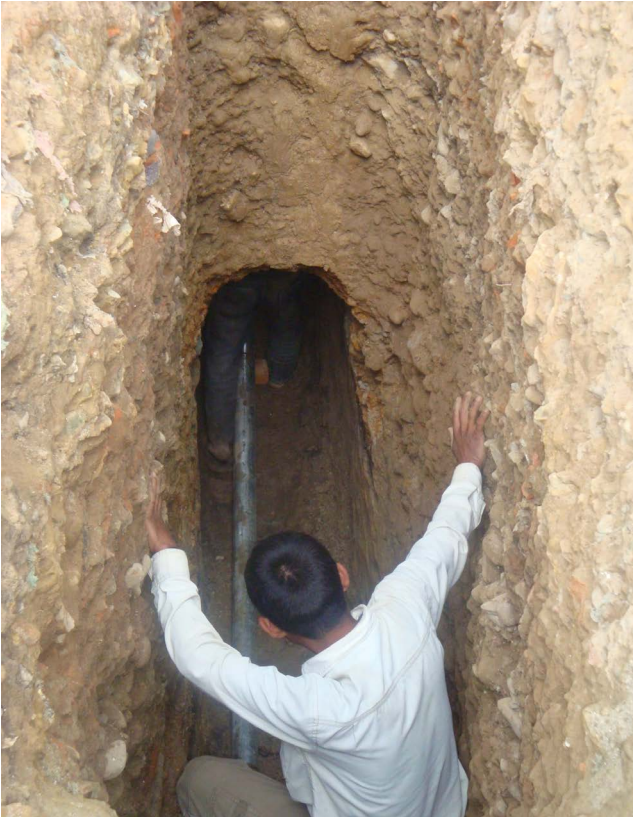
Installation of the new water line | 2015
