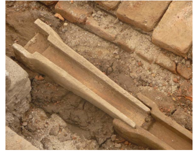
Historic water line The terracotta channel dating from the 17th century was restored and brings water from the original sources.
