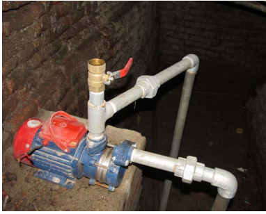
Underground pump house with a 1 HP pump installed
