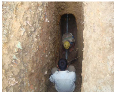
Tunneling under the East wing The new water line was installed at a depth of 3 meters.
