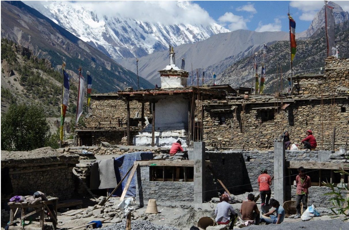
Figure 22: Construction site with stupa under renovation in Manang.
